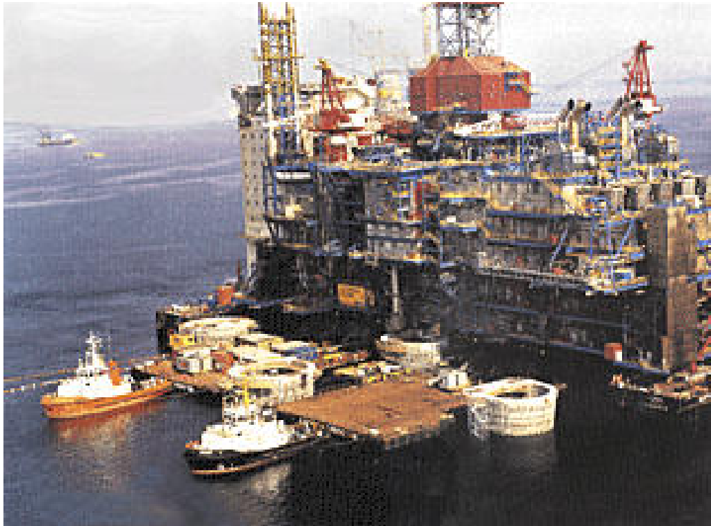
Figure 1.2: Sleipner A offshore platform under construction
